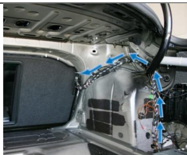
Figure 26 Cables are routed over the rear lid strutt.
